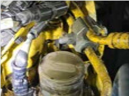
ELECTRICAL EMERGENCY ASSISTANCE
